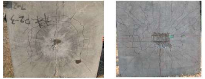
Fig. 3. Slab 10 after explosion, (a) upper face and (b) bottom face [31].
