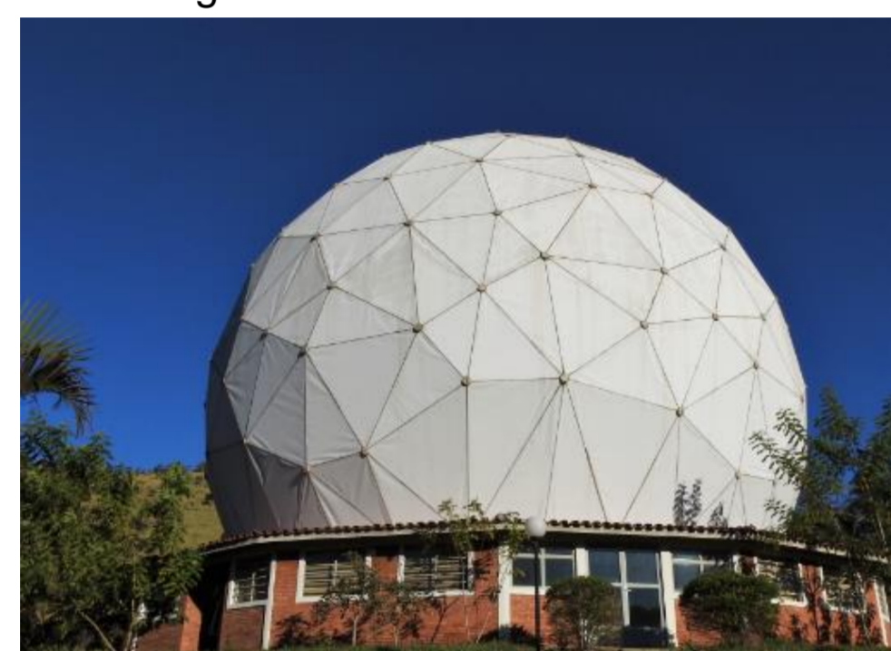
Figura 01 – Radome do RTPK.
